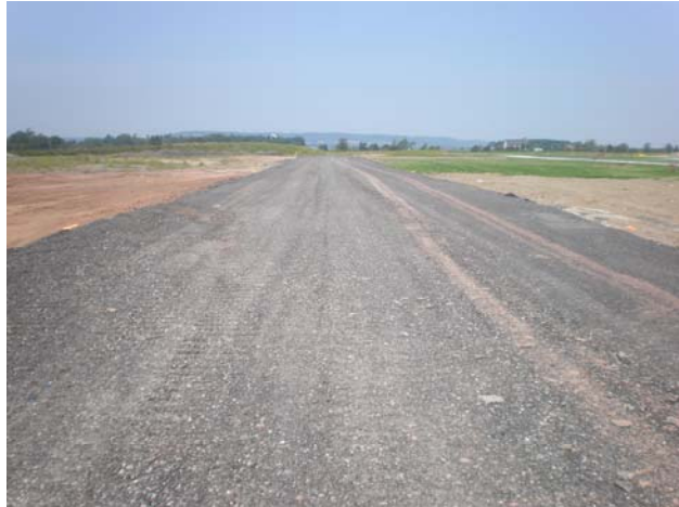
New laid out west taxiway looking north
