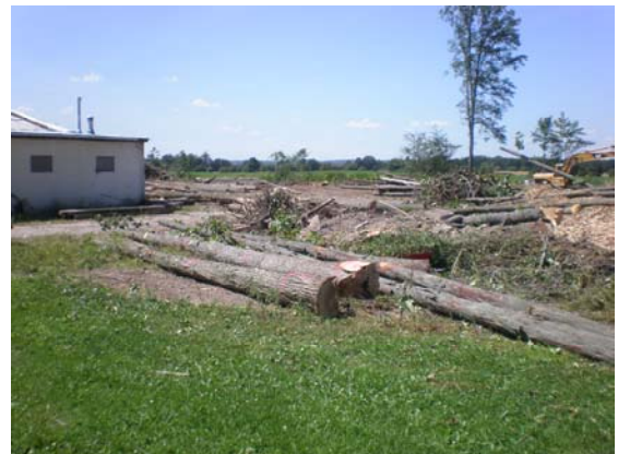
CLEARING WORK BEHIND THE PAINTSHOP
