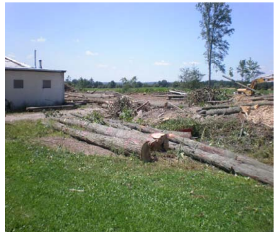
CLEARING WORK BEHIND THE PAINTSHOP
