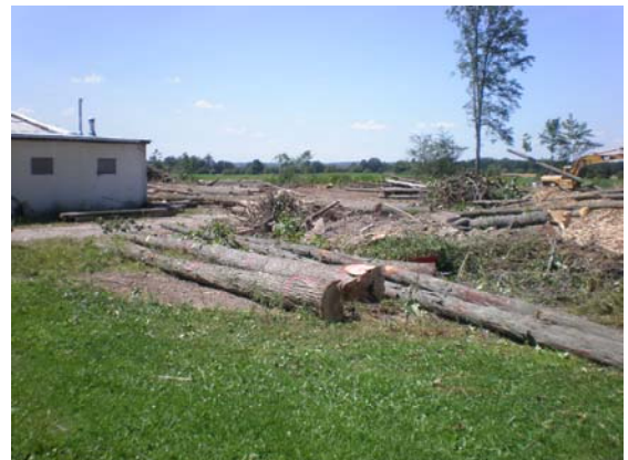
CLEARING WORK BEHIND THE PAINTSHOP
