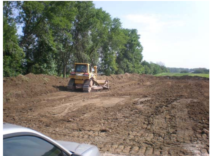
WEST SIDE WORK
