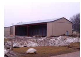
More work underway
