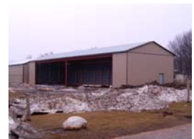
More work underway
