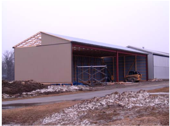
HANGARS ARE RISING UP AND WILL BE READY SPRING 2007
