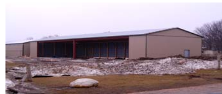
More work underway
