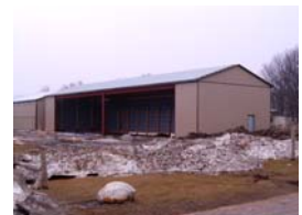
More work underway
