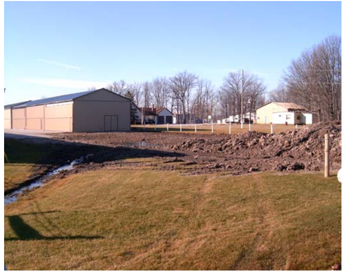
GROUND PREPARATIONS ARE UNDERWAY FOR CONSTRUCTION OF NEW HANGARS
