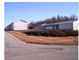
More work underway
